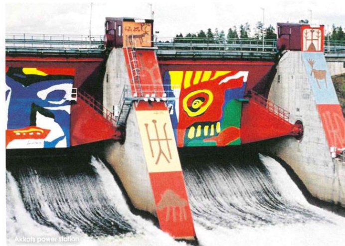
Akkats power station
